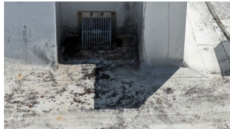
Maintenance Rooftop Drains
